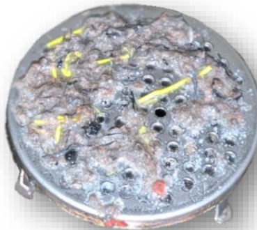
Figure 27 – Clogged Pump Intake Screen
